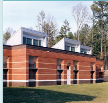
Figure S4.2 South-facing monitors.
