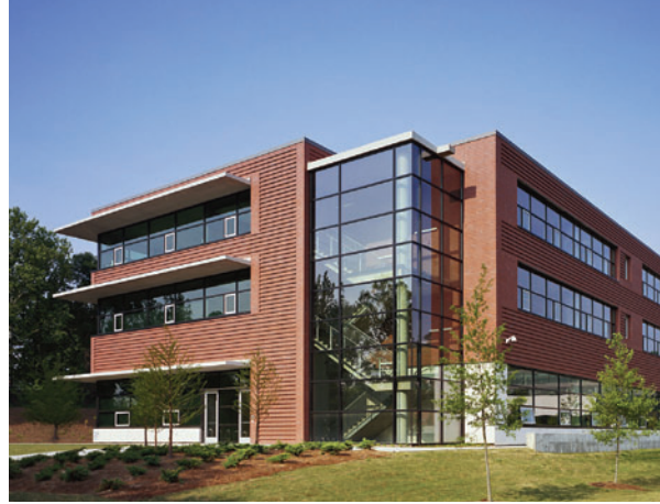
Figure 4.7. Building exterior with light shelves.
