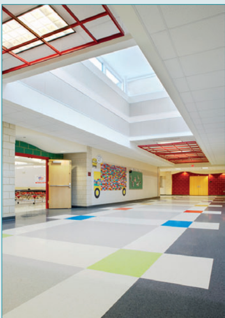
Figure S2.1. Corridor daylighting.
