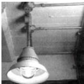
Typical Class 1 Div 1 conduit installation
